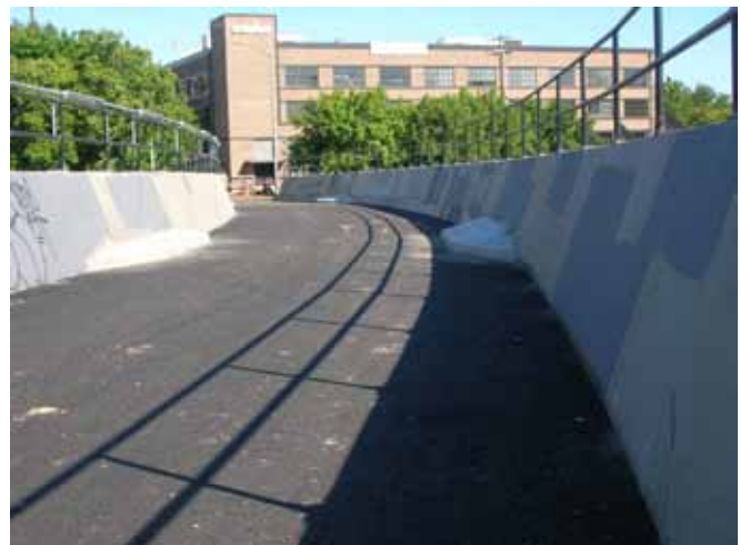
Top: The prize-winning mobile bike service station. Photo by Mellissa Meng. Bottom: The R Street bridge in August 2009 just before it was striped and officially opened for traffic. SABA file photo
